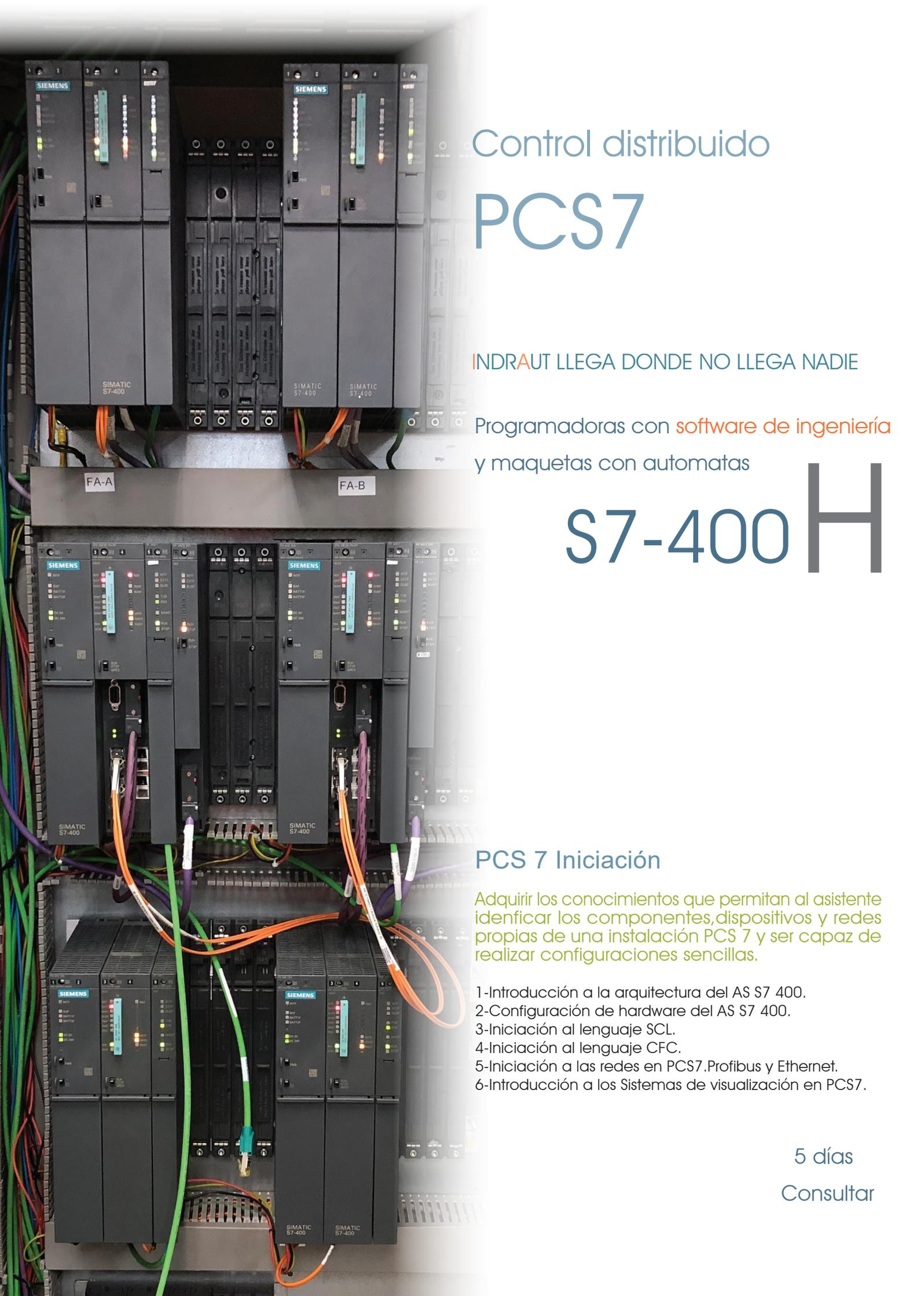
A photograph of a Siemens SIMATIC S7-400 PLC rack. The rack is filled with various modules, including power supplies, CPU units, and communication modules. The units are labeled 'SIEMENS' and 'SIMATIC S7-400'. The rack is divided into two sections, FA-A and FA-B. The background is a light, hazy gradient.
